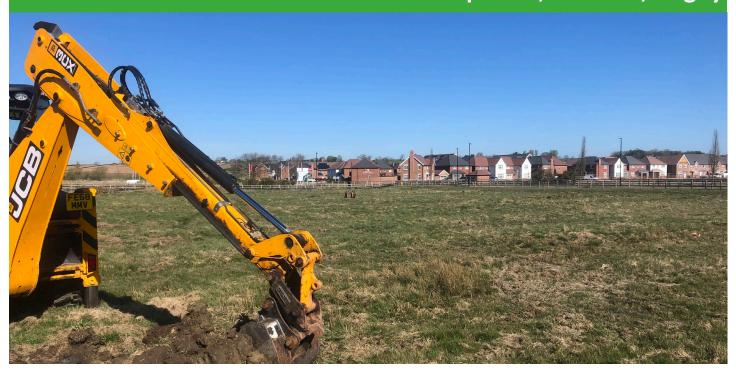
JPP Geotechnical and Environmental were appointed to undertake a supplementary geotechnical ground investigation to assist our in-house structural engineers on a prestigious residential project in Houlton. Our geotechnical design team specified and undertook a parcel-specific supplementary geotechnical ground investigation using trial pitting techniques to allow the refinement of the proposed foundation solutions on a plot-by-plot basis.
